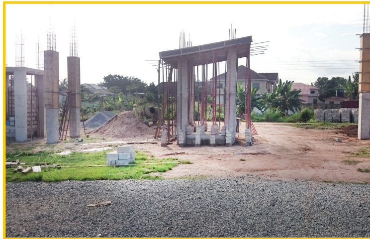
Construction of Security Gatehouse at college entrance
