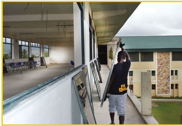
Construction of 3rd floor classroom wing
